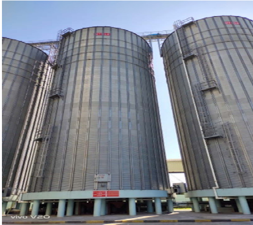
Grain Silo Area
